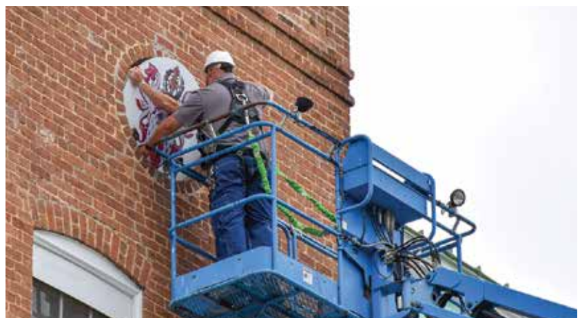
At left, Commandant of Cadets Maj. Gen. Randal Fullhart removes the weathered heraldry from Lane Hall. At right, university workers replace it with a new Corps shield done in metallic colors.
