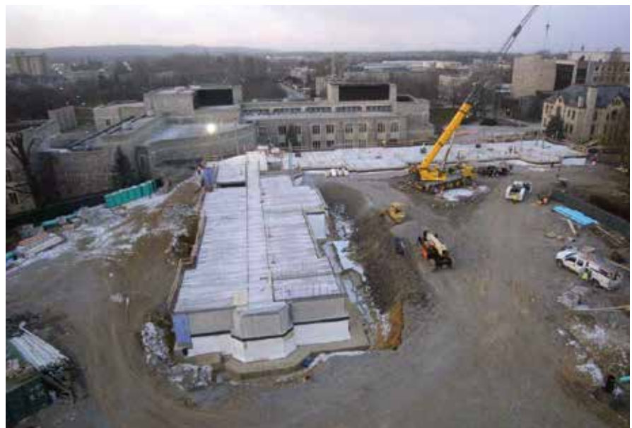
Construction of the Corps' second new residence hall for cadets has begun.
