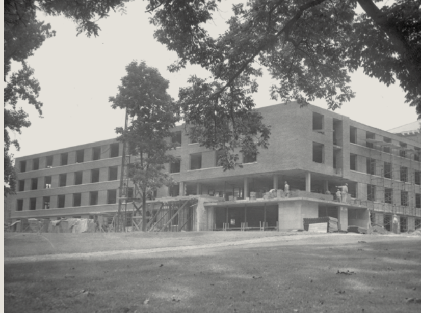
Construction of the "new" addition in 1957
