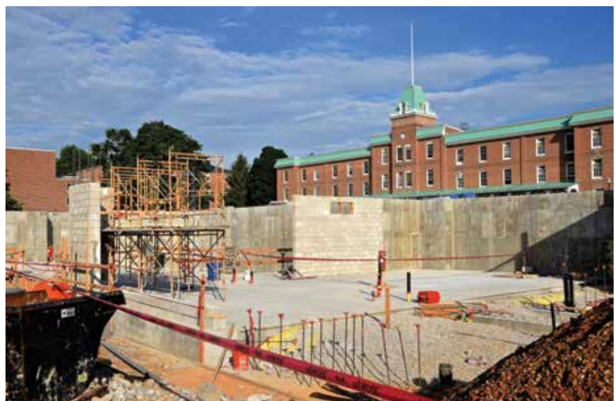
The walls of the Corps' new dorm on the Upper Quad are rising.
