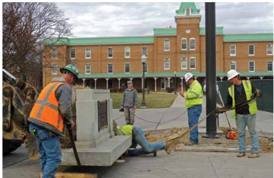
Workers relocating the Corps’ monuments and cannons to a temporary location on the Upper Quad
